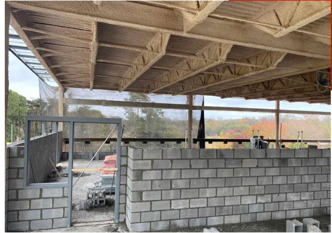
CMU Progress at 4 th Floor of New Addition
