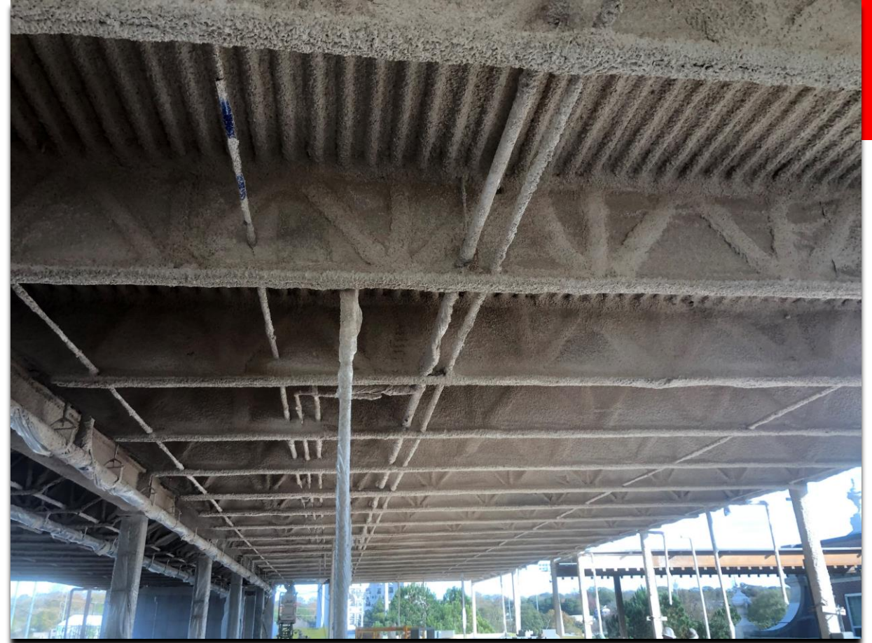
Fireproofing Complete at New Addition
